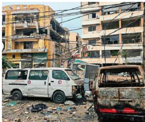
Damaged buildings and vehicles in Beirut after an Israeli airstrike, on March 21. The Israeli military said it had launched strikes targeting Hezbollah. AFP
